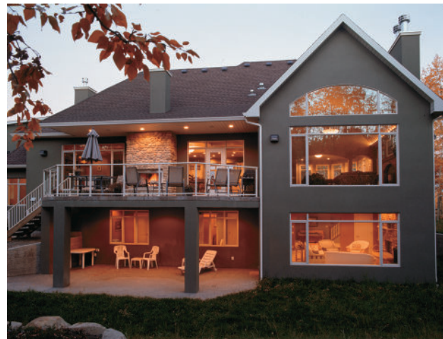
Areas under balconies, decks and porches that are clear of debris can limit the effect of a wildfire
