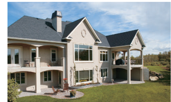
Stucco is a siding material that can be used as it offers fire resistance.
