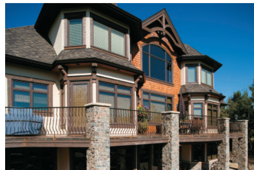
Wooden shingles can be used as a decorative element as long as it is not the main material used for exterior siding.
