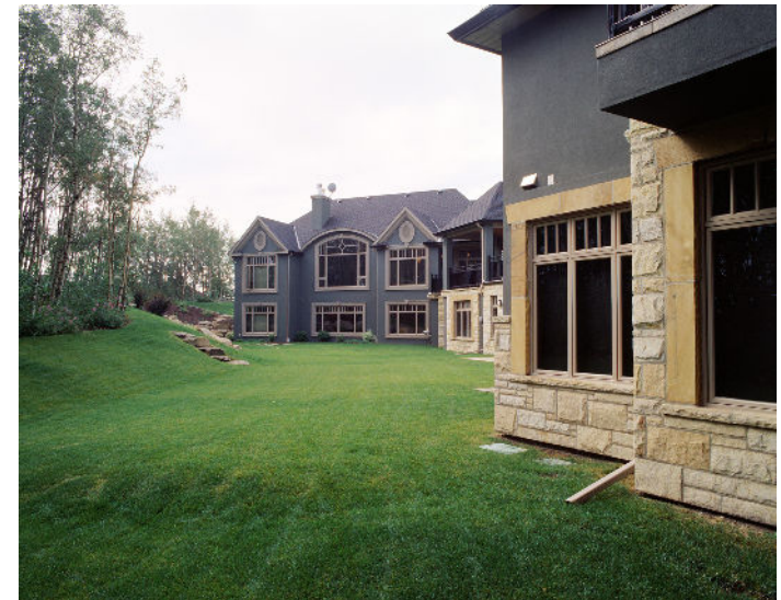
Removal of flammable vegetation within 3.0 metres of a structure will assist in minimizing the effect of a wildfire.
